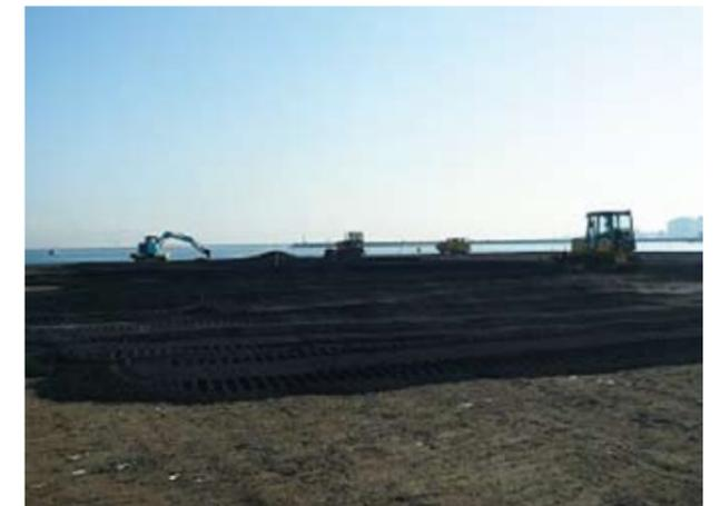
Construction using Reglobe as a sand-blow prevention material
